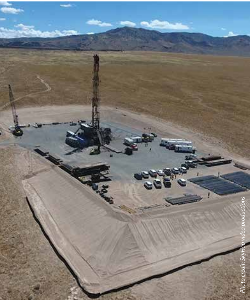
View looking east toward the Mineral Mountains, during the drilling of well 58-32, the initial test well at the FORGE site. The well reached a temperature of 199°C. at a depth of 7536 ft.
